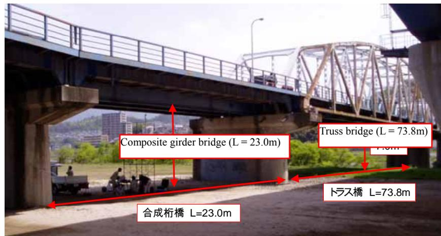
Fig.11: The Composite Girder and Truss Bridges.
